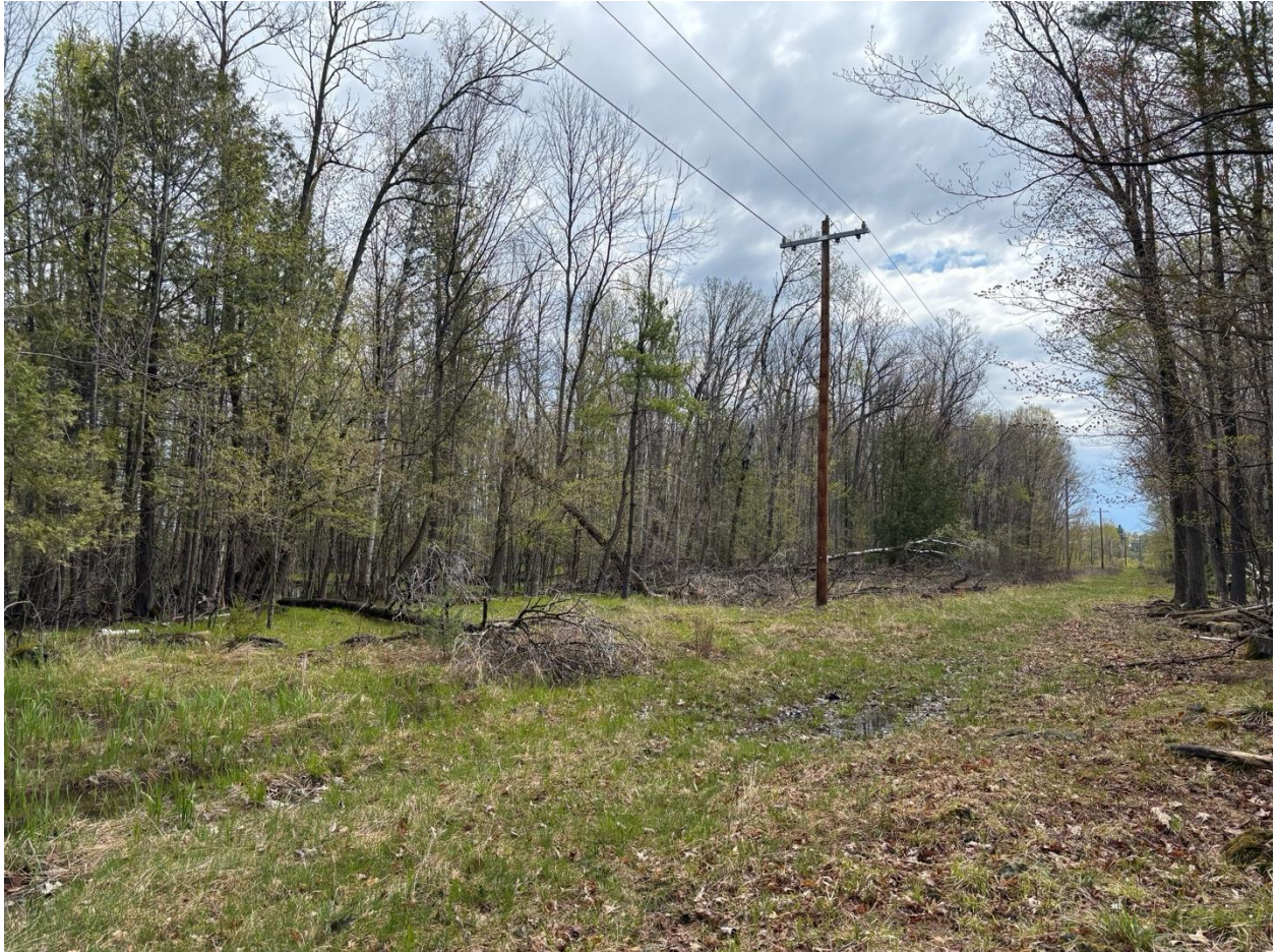
Photo taken outside of AOI, north of UDP-2, facing a northeasterly direction along high line.
